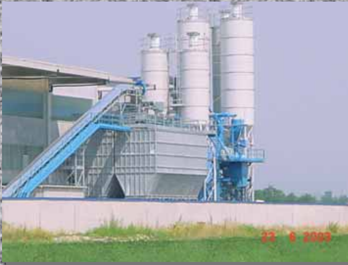
Plant for production of pre-cast panels.
